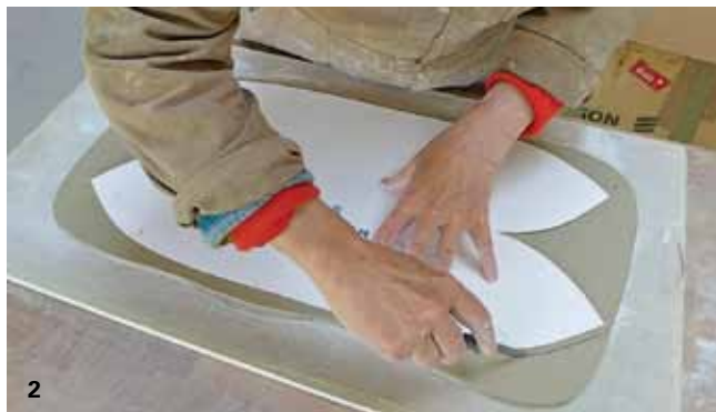
2 Cut the slab approximately 1/2-inch larger than the cardboard template. Bevel the V-shaped ends at a 45° angle.
